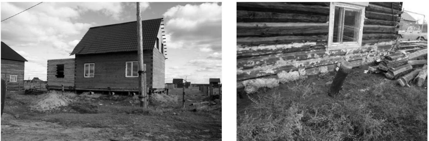
FIG. 5. Two methods of protecting permafrost: (left) by creating an insulating layer under new house construction and (right) by retrofitting existing buildings. Churapcha region, Central Yakutia (photos by A.N. Fedorov and P.P. Fedorov).
